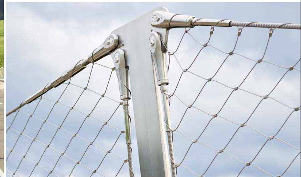
Hundwilertobelbrücke, Appenzell AR (CH)
